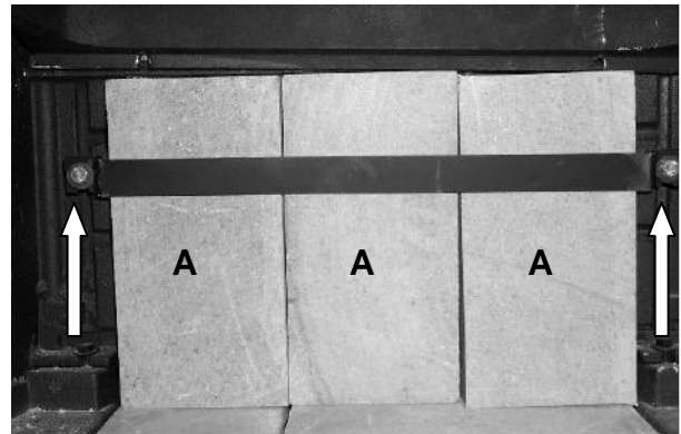
Photo 14 – Install & Secure Firebox Rear Stones
