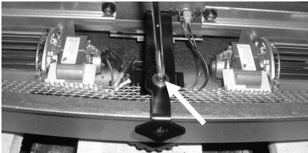
Photo 26 – Air Control Mounting Detail
